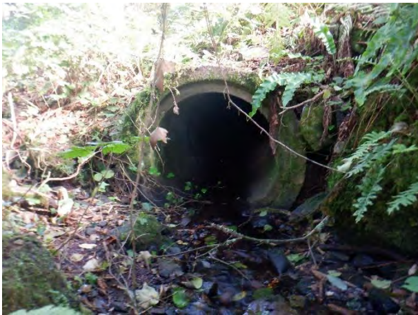
Plate 4-11: Glasheen as it enters the second pipe under the Bandon Road.
