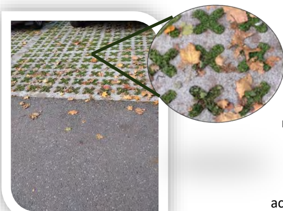
Figure 8-6: Example of green paving solution in the car park at the Marina in Cork City.
