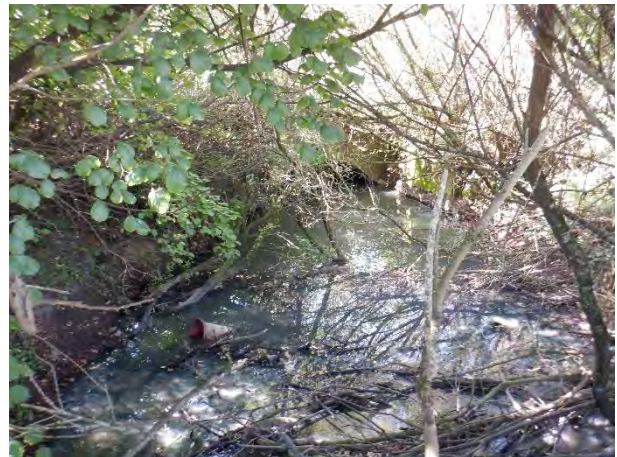
Plate 4-25: Glasheen as it emerges from the culvert under Sarsfield Road.
