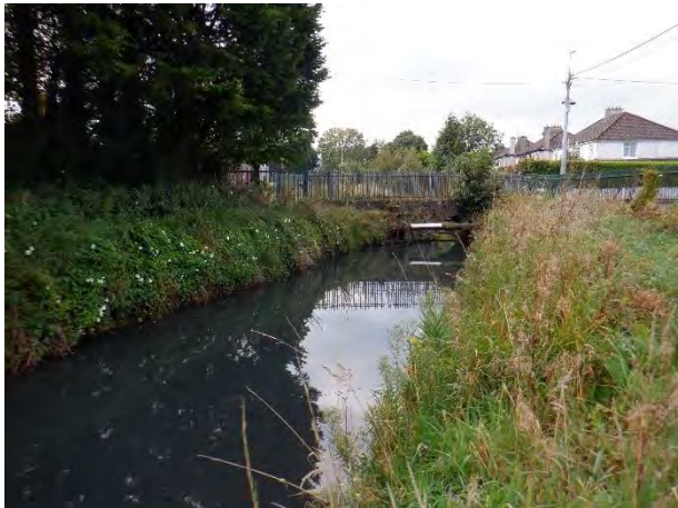
Plate 4-28: Glasheen at Site 6 looking upstream at the pedestrian bridge.
