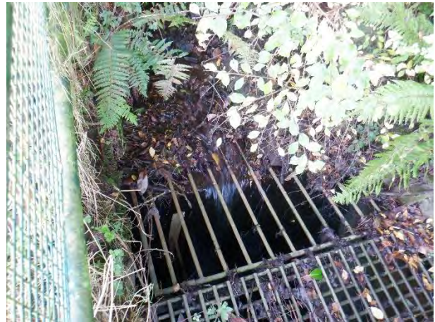
Plate 4-2: Glasheen as it drops 1m down a concrete ledge and piped under the cemetery.
