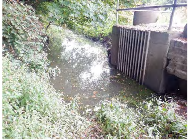
Plate 4-33: Glasheen at Site 7 as it enters the culvert diverting it under Magazine Road.
